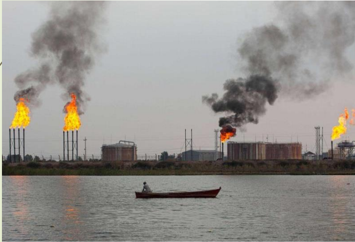
Figure. The flares in the refinery
